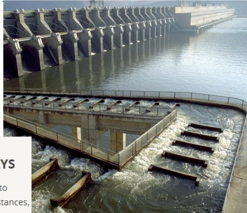
Fish ladder built around a dam in the Pacific North West. Harald Sund/Photographer's Choice/Getty Images
