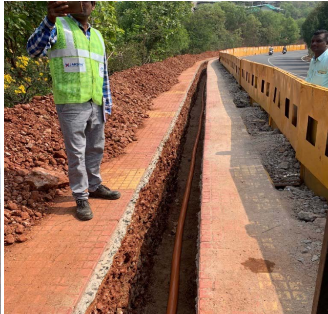
ANDHRA PRADESH UNDERGROUND CABLING
